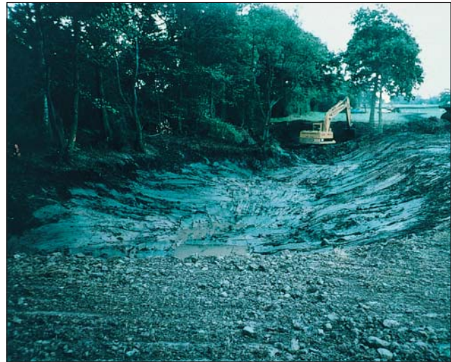
A 19th century origin Cheshire farm pond, used as a rubbish dump for thirty years, has been excavated in autumn, to its original shape
